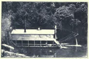
Photo lent by Leo Weinthul A STEAM DREDGER AT WORK IN A GOLD COAST RIVER, EXTRACTING THE GOLD FROM THE SAND AND MUD OF THE STREAM
